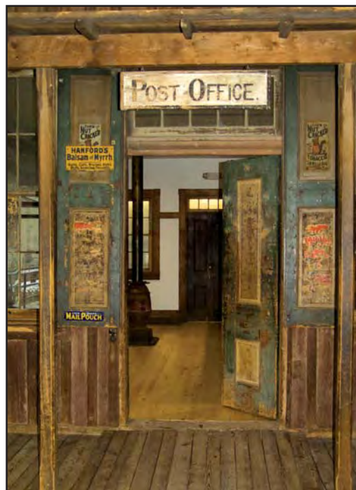
The entrance into the Headsville Post Office.
