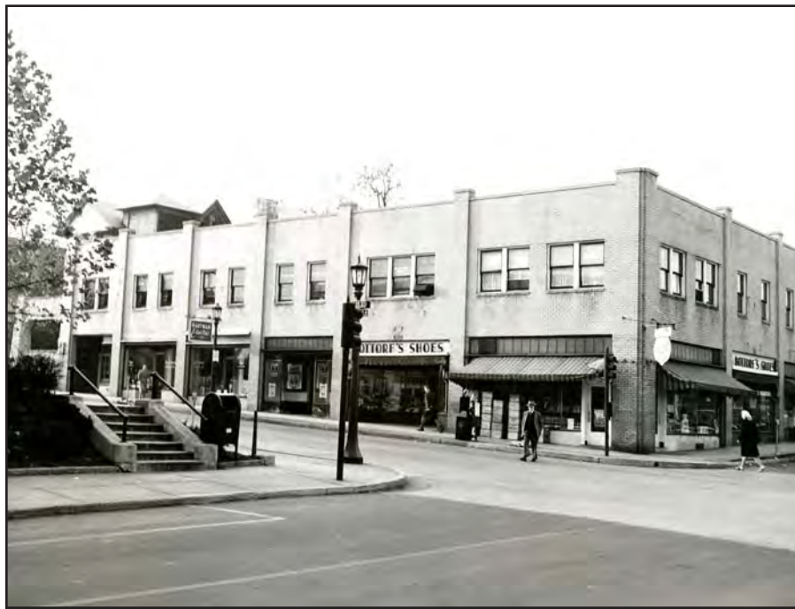
The first APS located in State College, PA, was located on the second floor of this building.
